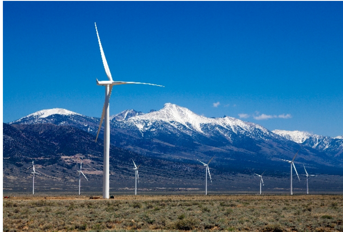
Spring Valley is a 152 MW project located in White Pine County, Nevada. The project consists of 66 2.3 MW turbines that commenced commercial operation in August 2012.
