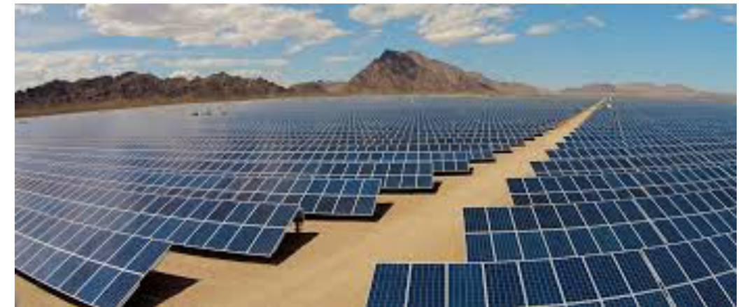
The Copper Mountain Solar 3 project in Boulder City, Nevada (250 MW capacity).
