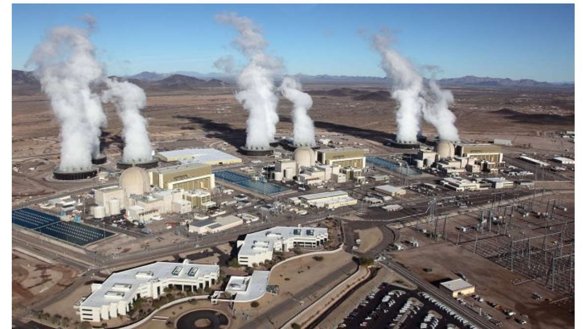
Palo Verde Nuclear Generating Station, Arizona
